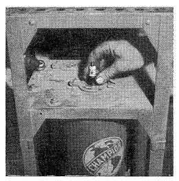
& Remove and clean spark plugs. The mechanic is shown cleaning a spark plug in the SE-861 spark plug cleaner. Plugs having burned electrodes or broken porcelains should be discarded. Blistered porcelains indicate that the wrong type plug is being used and a change of heat range should be made.
